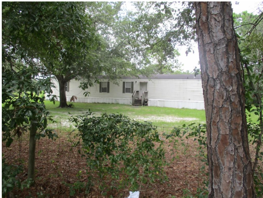
View of a structure on the subject property along Noroad.
